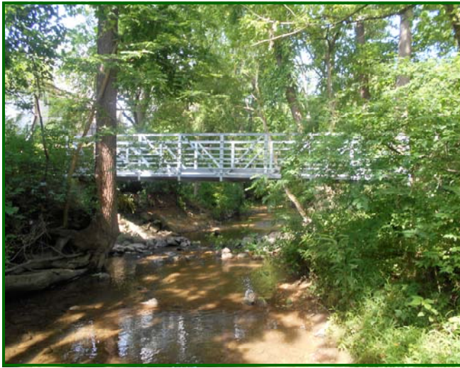
New downstream bridge.
